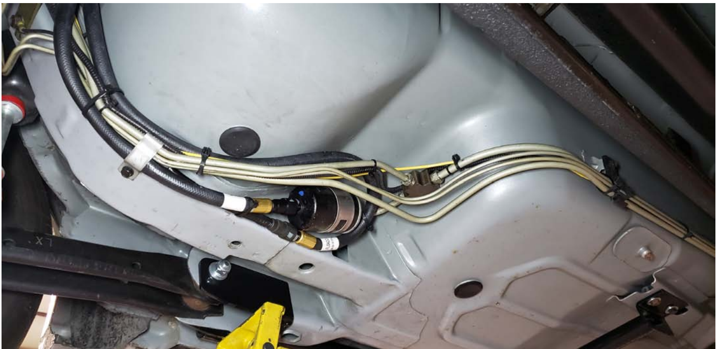
Fuel Pump Lines Installed
