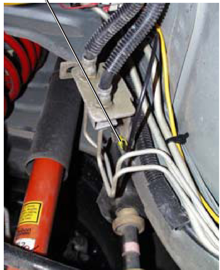
Fuel Pump Ground Mounting Location
